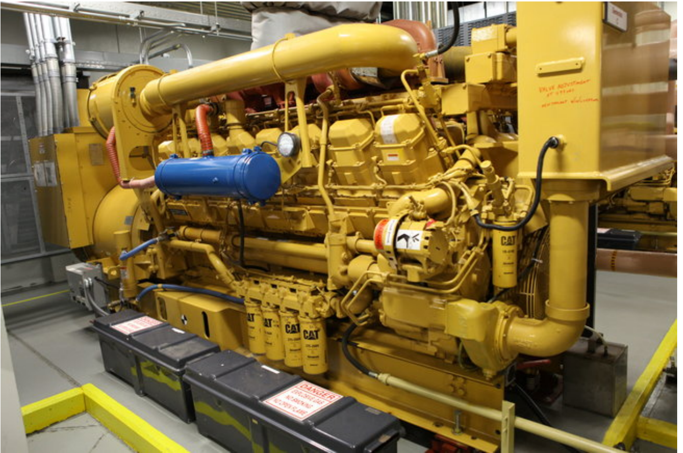
A backup diesel generator at a large computer data center, one of six in the room. Combined, they could provide enough power for a community of 7,000 homes. (NY Times)
